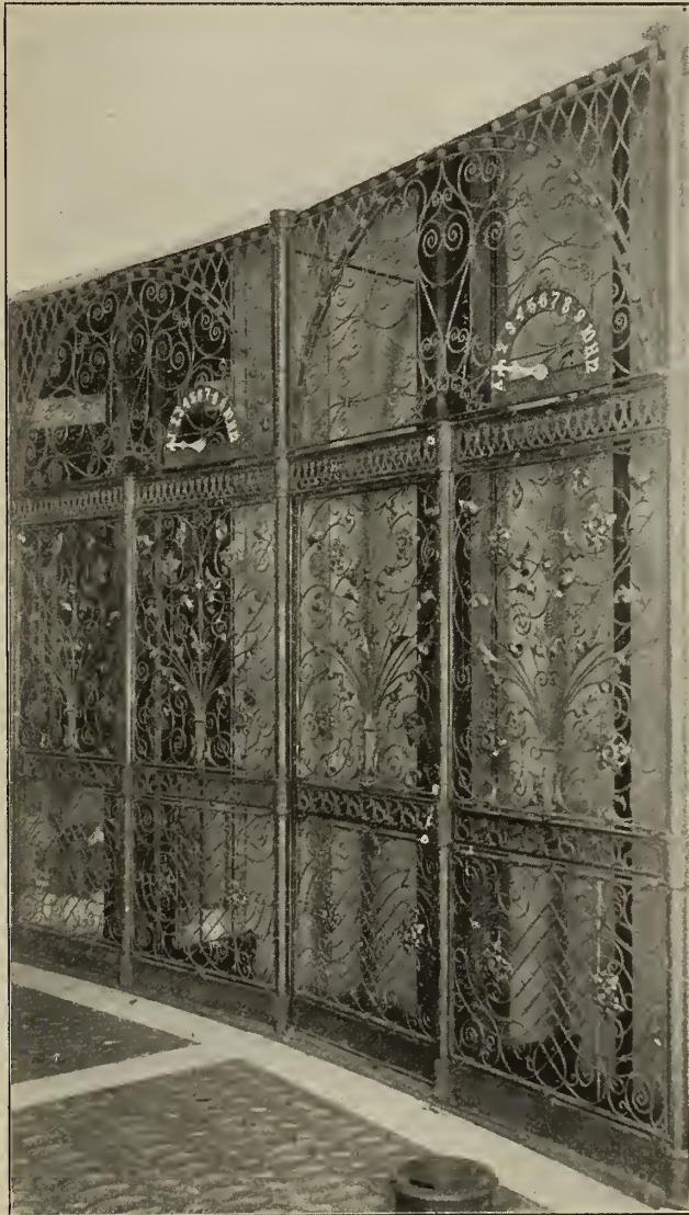
A.—ELEVATOR INCLOSURE, THE WOMAN'S TEMPLE, CHICAGO. Wrought Iron, Hammered Leaf Work
